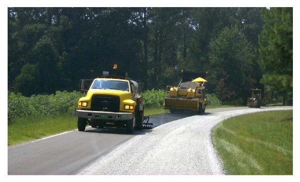
Figure 20. Asphalt distributor followed by the stone spreader and roller.
