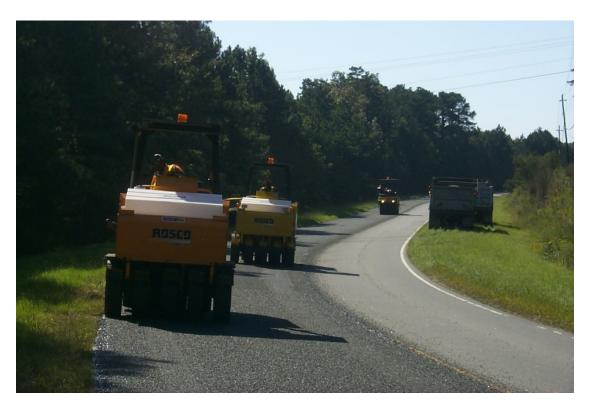
Figure 21. Two pneumatic tire rollers followed by a static steel wheel roller or combination roller.
