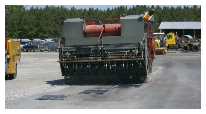
Figure 13. Calibrating the stone spreader.
