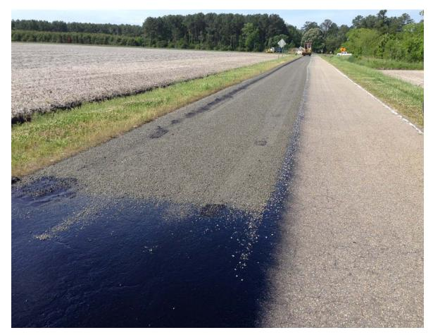
Figure 26. Insufficient Aggregate.
