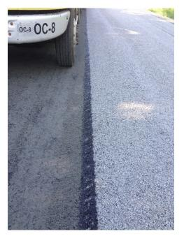
Figure 28. Centerline Tie Strip – Longitudinal Joints.
