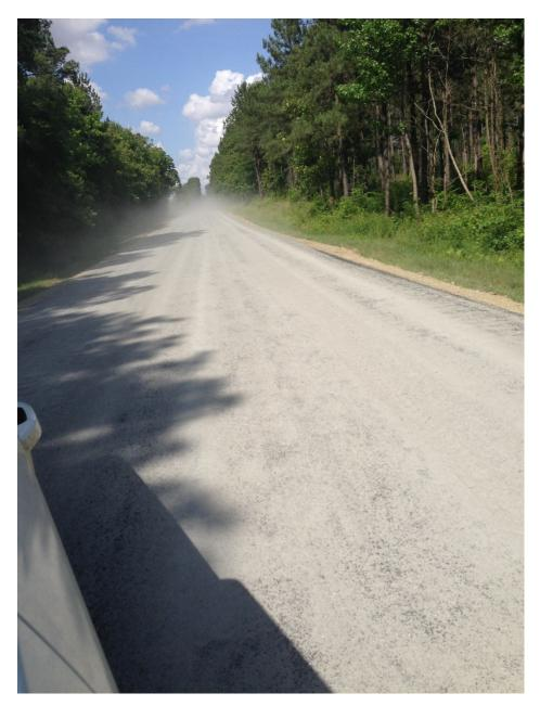
Figure 27. Excessive Aggregate.
