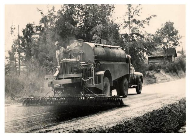
Figure 1. Road Oil in North Carolina in 1942; courtesy of E.D. Etnyre & Company.
