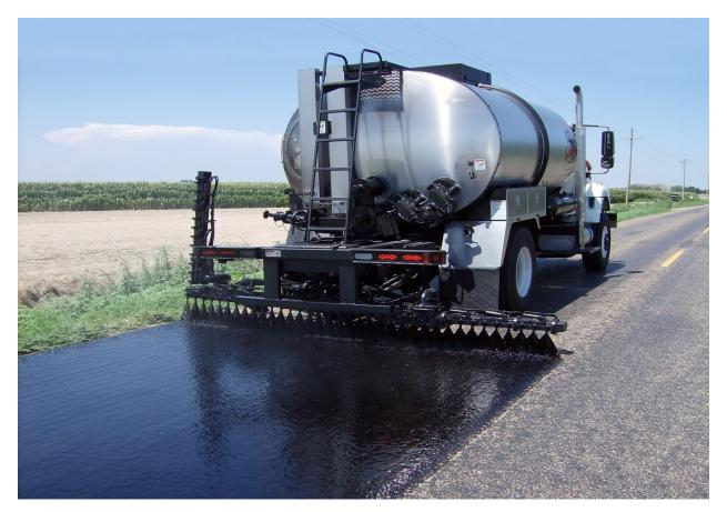
Figure 5. Asphalt Distributor operating at the proper spray bar height to apply double coverage; courtesy of E.D. Etnyre & Company.
