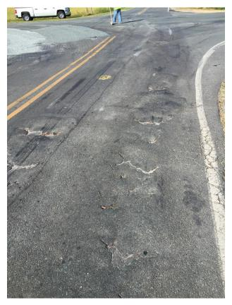
Figure 4. Severe Alligator Cracking.
