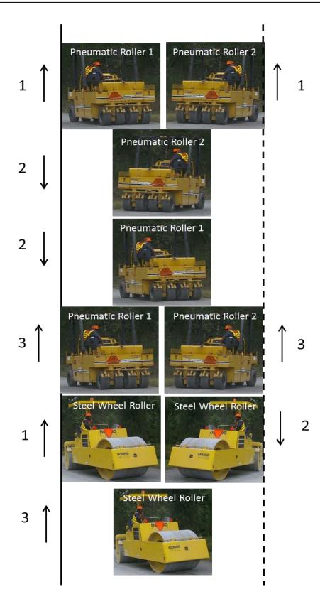
Figure 22. The rolling sequence on the first side of the road.
