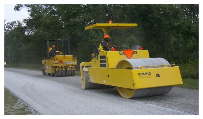
Figure 8. Pneumatic tire roller (in background) being followed by static steel wheel roller (in foreground).
