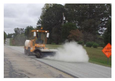
Figure 10. Mechanical broom operation.
