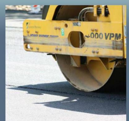
1<sup>st</sup> pass all on hot mat with roller edge off joint approx 6-12 inches
