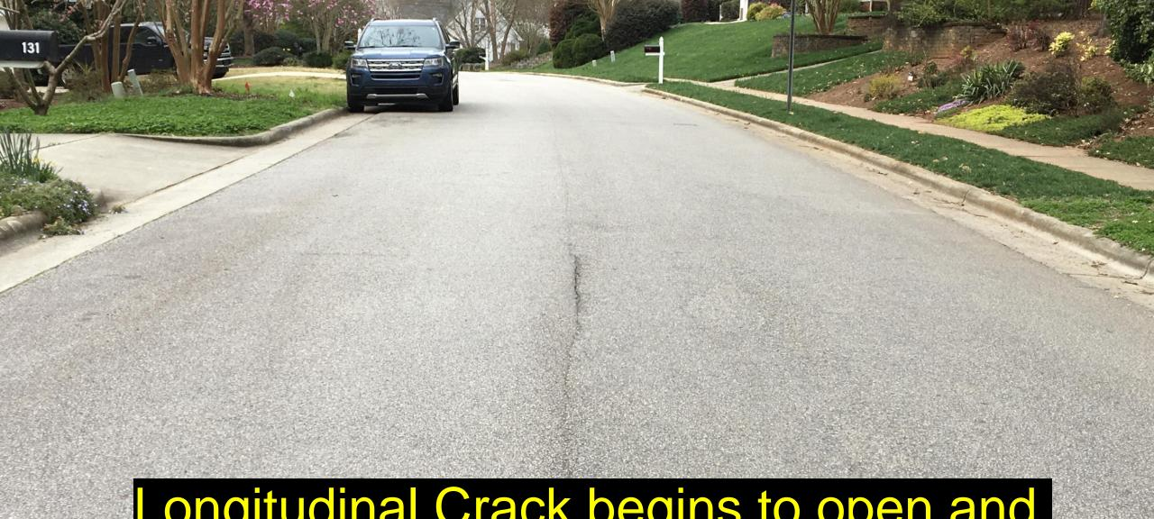
Longitudinal Crack begins to open and allow water into the pavement
